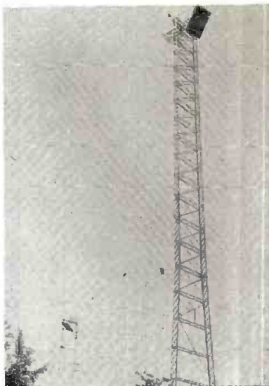
THIS is new two-tower array of the Bell microwave relay system completed for WJIM-TV Lansing, Mich., and part of the $250,000 Bell system completed by AT&T. Signal is beamed from Detroit to 274-ft. tower at Milford, to a second tower at Danville, to receiver in Lansing and then to the WJIM-TV tower.
